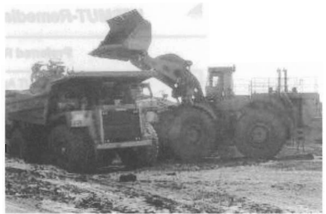
Photo2 Reclamation of Paitzdorf Waste Rock Dump, Ronneburg Site
