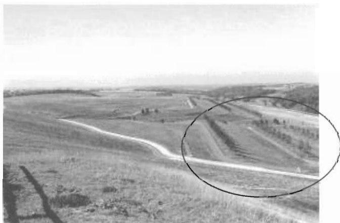
Photo6 An Example of Revitalization of Ex-uranium Mining Area at Ronneburg Site
