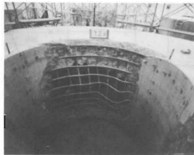
(1)Blasting of Thin Layer Reinforced
