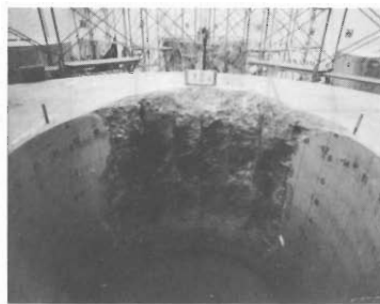
(2)Blasting for Loosening of Thick Layer Non-Reinforced
