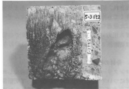
Photo 5 Cut Surface of Concrete Specimen with D 41
