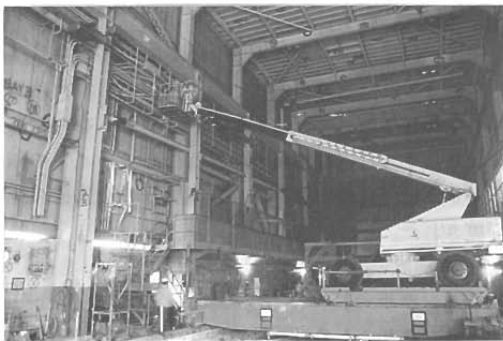
Photo 7 Decom worker in a man-lift in the FHB (Ref. 213/18)
