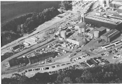
Photo 1 SSDP site status prior to commencement of physical decommissioning (Ref. DOE/SSDP-0081)
