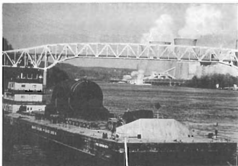
Photo 6 Departure of the loaded barge from the Shippingport Site (Ref. 322/24)
